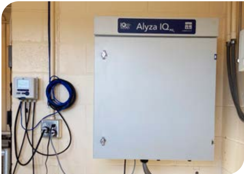
The Alyza IQ PO4 analyzer installed indoors in the UV disinfection building, providing continuous orthophosphate monitoring.
